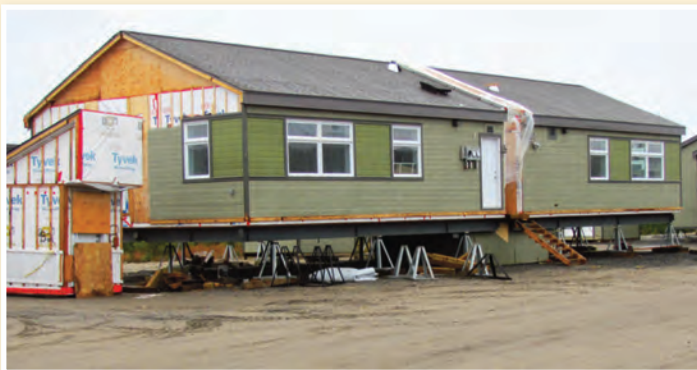
Semidetached homes under construction in Kuujuaq, 2010.
